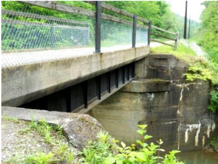
1924 in concrete of both abutments
