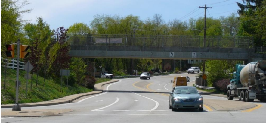
View from Valley Brook Road intersection. Thomas Road is the left turn beyond bridge.
