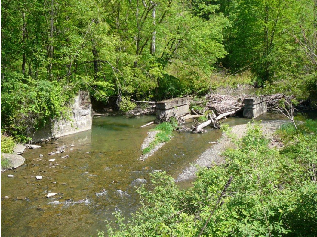
Old abutments on original Right-of-Way carried a 3 span bridge.
