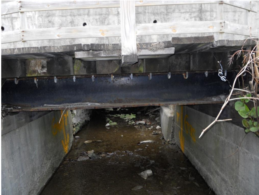
This view of Main Line span in 2010 – No Builder's Plate – welded steel construction
