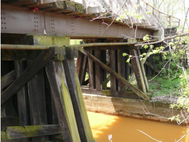
3 sections of I-Beam spans on timber bents.
