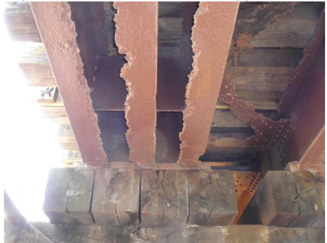
Triple I-Beams on each side to support rails
