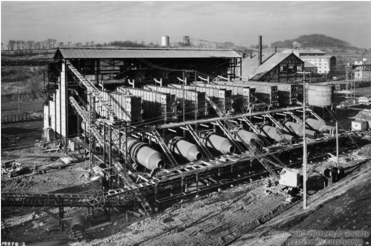
The carbonization process also produced gases and coal tar. The gas was recycled into the DISCO plant furnaces as a fuel and the coal tar was stored in large tanks and sold to the Koppers Chemical Company, a major producer of chemicals made from coal tar. A ton of coal could produce 1,440 pounds of DISCO, 3,400 cubic feet of fuel gas, and 15 gallons of coal tar.
