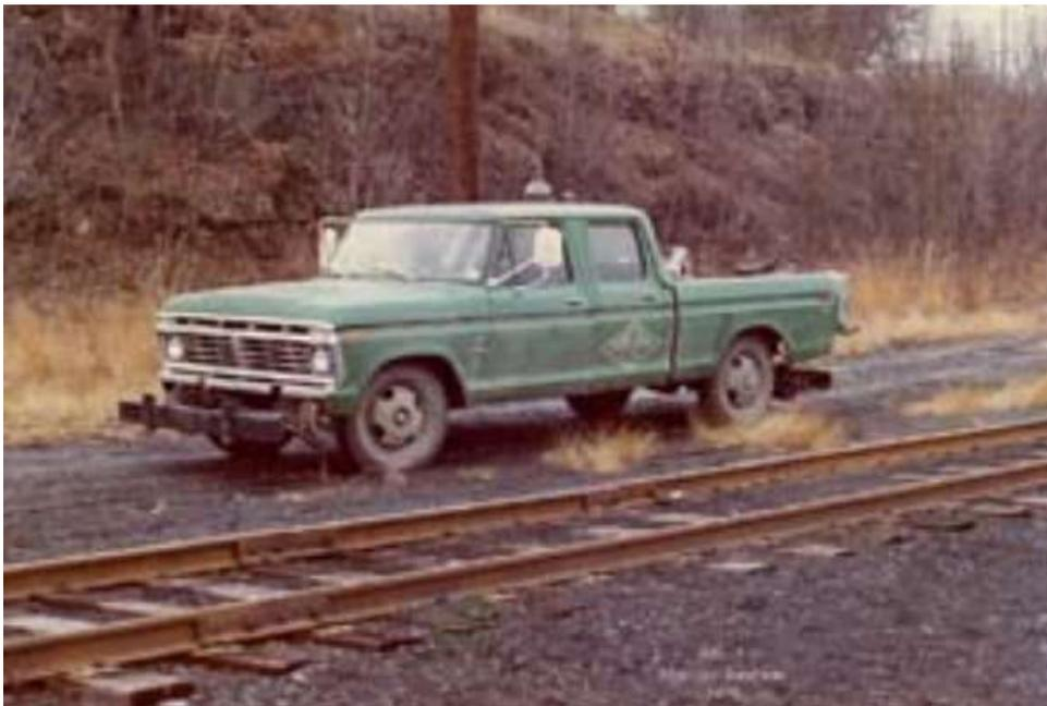
The maintenance trucks were Ford hi-railers [a truck that can operate on both highway and rail]. Gene Schaeffer provided this 1975 photo of RH-1 taken at Montour Junction, which was used by Section Gang 1 and kept at the Champion Yard. Tim Sposato's RH-2 was kept at Hills Station. Photo courtesy of Gene P. Schaeffer ©2012
