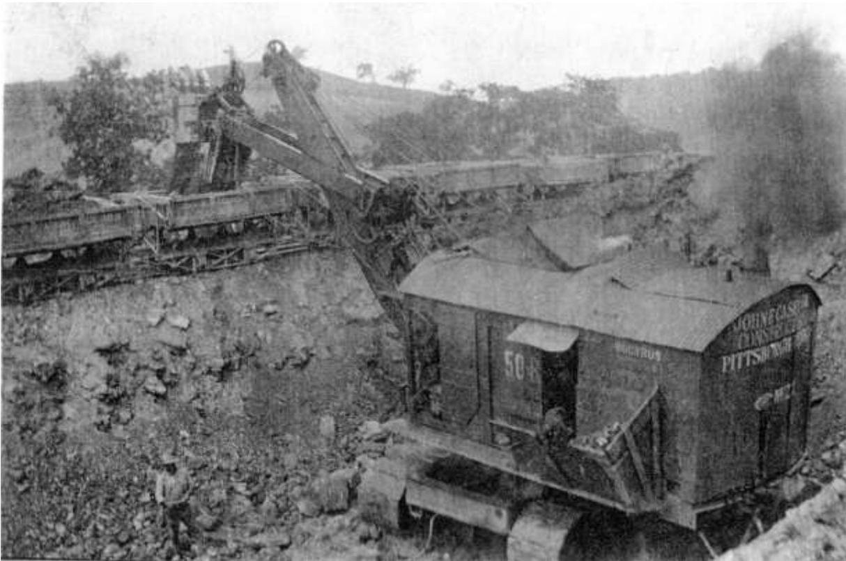
After the train of side-dump cars was loaded, it was hauled to the Hutchinson farm where it was used to create a high fill to keep the grade as level as possible. Note the flimsy looking temporary trestle used for the dump train. The timber was left in place and buried under the fill.
