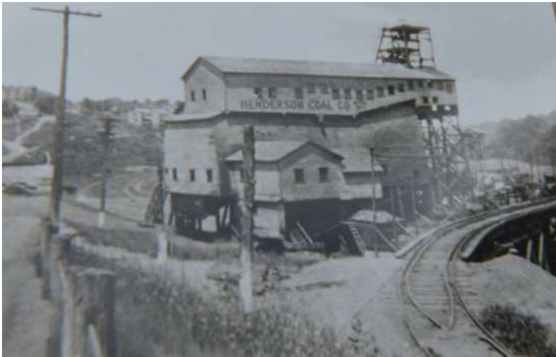
The Henderson Mine tippie building. The tracks at lower right carried larry cars to the waste dump across Morganza Road. Photo courtesy Paul Katrencik.
