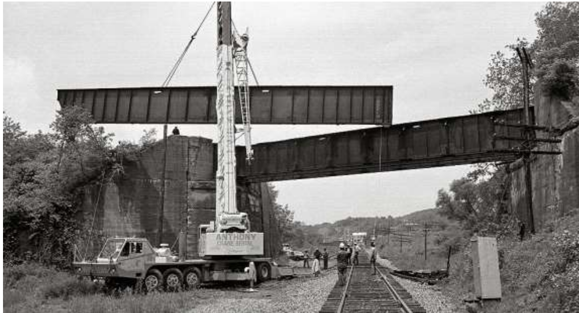
The bridge carrying the Montour main line and siding over the N&W railroad near Baptist Road is removed June, 1981. Gene P. Schaeffer photo.
