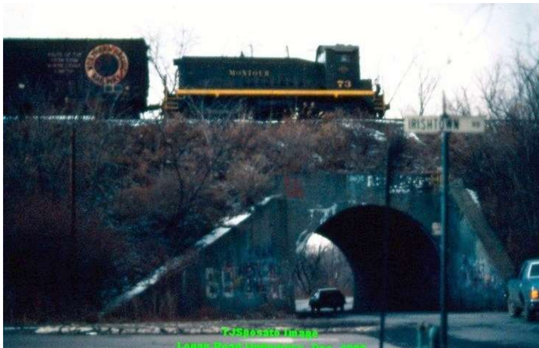
One of the last trains to Brookside Lumber crosses over Logan Road in December 1980. The concrete arch bridge was demolished in 1987. Tim Sposato photo.
