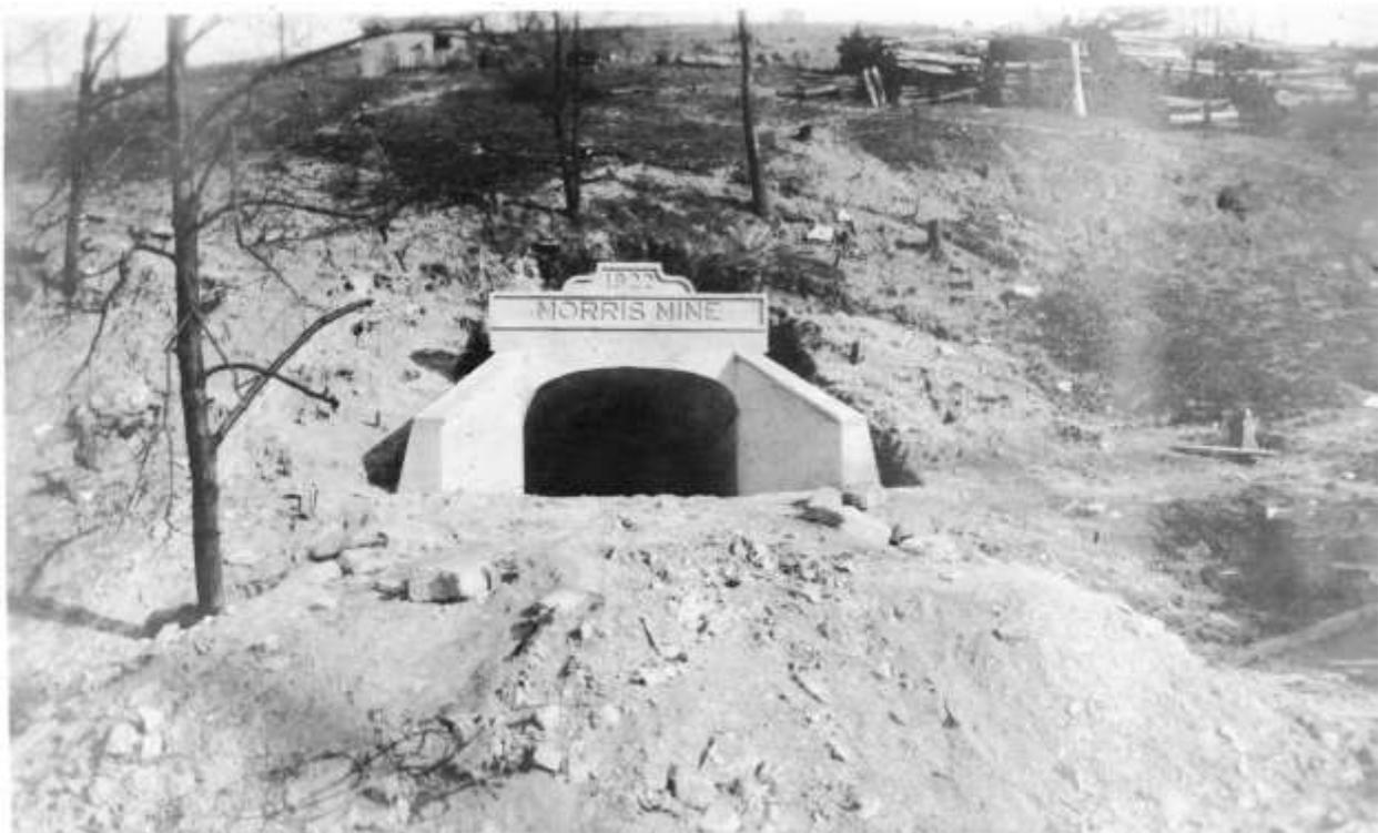
**Men and supplies entered the mine using tracks laid into the sloped shaft at this portal. The waste dump would grow on the hillside above the portal.**
