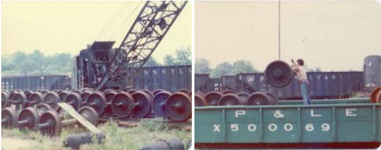
X1 unloads wheelsets at the Montour Junction car shops.
