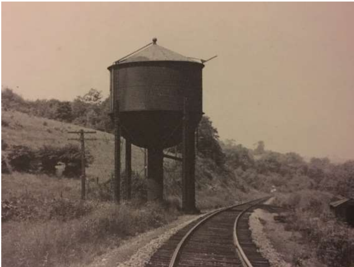
The steel Fife water tank sits beside the main line in the 1920's. Concrete footers for the four legs and the central column can be found near the edge of the trail. Photo from Gene P. Schaeffer Collection.
