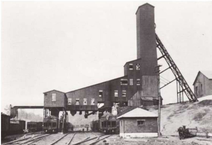
Loading tippie at National Mine No. 3 in Muse, PA. Photo courtesy U. S. Steel Company
