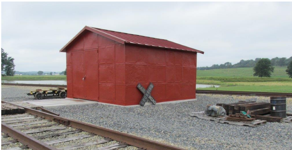
Salvageable pieces of three original sheds were used to reconstruct a Montour tool house at the Age of Steam Roundhouse. Tim Sposato photo
