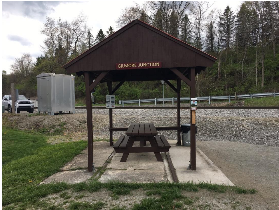
The tool house slab at Gilmore Junction shows rails imbedded in the concrete slab. Bryan Seip photo
