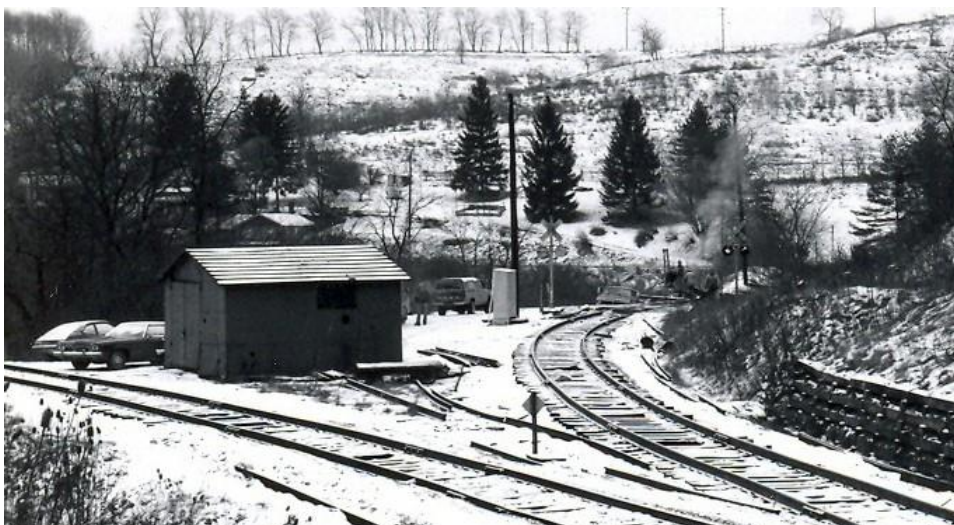
The tool house at Gilmore Junction is seen in this 1981 scene. The doors on the left side gave a motorcar stored inside access to the main line track. Tim Sposato photo
