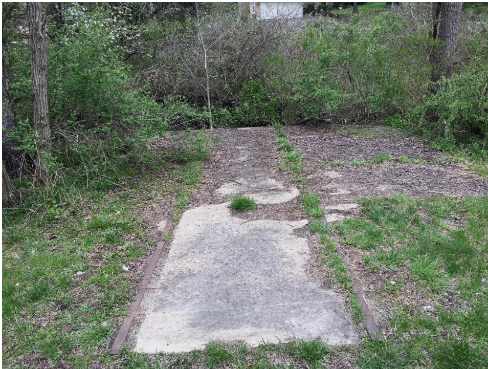
A weed covered concrete slab with rails embedded shows the former location of a tool house at trail mile 15. Bryan Seip photo.
