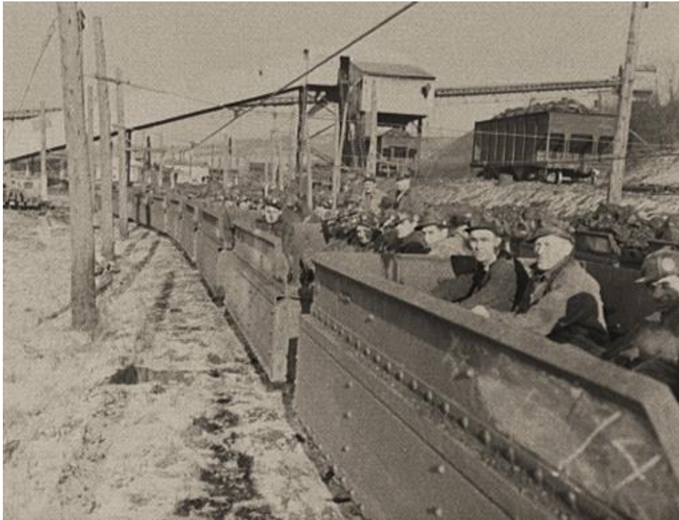
Miners crowd into mine cars at the start of their shift at Westland for the Man Trip to the working face inside the mine.
