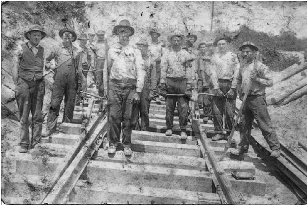
A track gang installs the east switch at North Star Junction near Imperial ca. 1913. Photo courtesy Andy Hanna / Kevin Kovach collection
