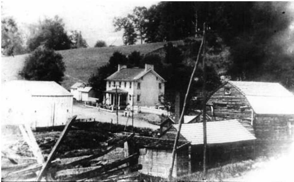
McPherson's Mill, ca. 1870. The Hendersonville post office was in the house on Morganza Road, which was razed in 2021.
