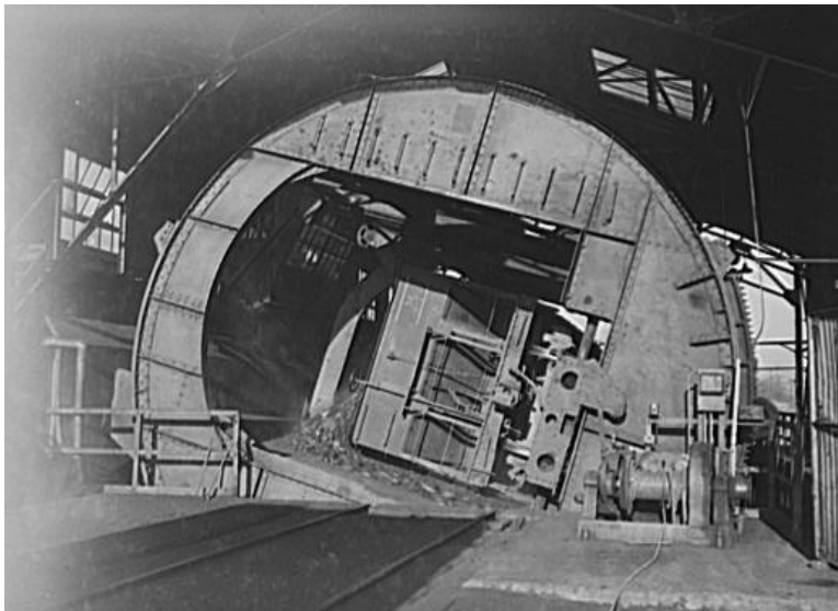
The rotary dumper flips an entire hopper car upside down to empty its load of coal. John Collier photo.
