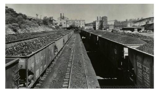
This view from the opposite side of the plant shows hoppers loaded with processed coal ready for shipping to final customers. Note the different textures and sizes of the coal in the hoppers.
