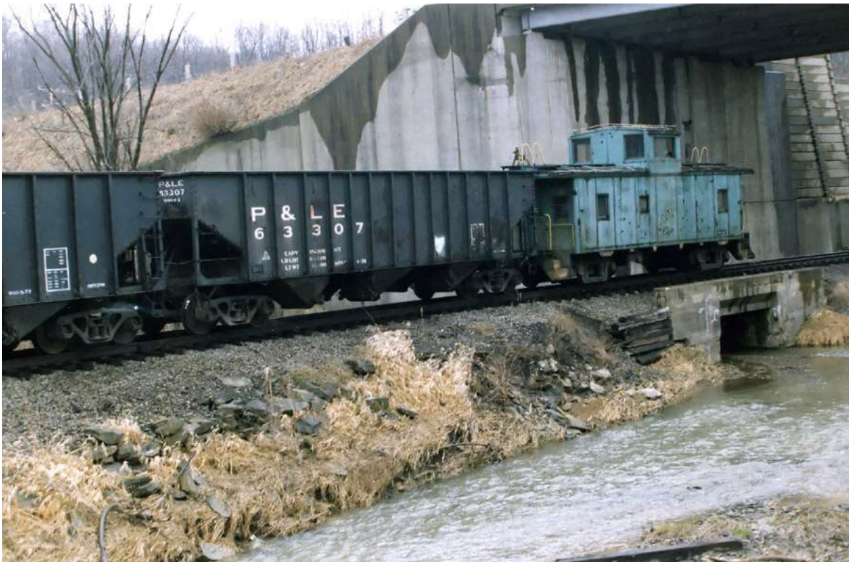
This short concrete slab bridge seen under the caboose crosses a stream flowing into Montour Run next to Beaver Grade Road.
