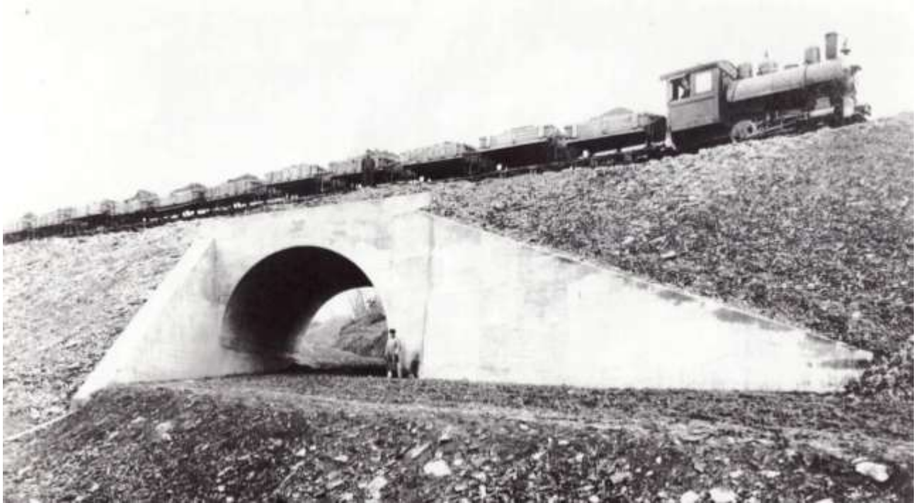
The concrete arch at Beagle Club Road was built in 1913 during construction of the of the Montour Railroad extension to West Mifflin. It is still in place today carrying the Montour Trail. Photo courtesy Dave Richards.
