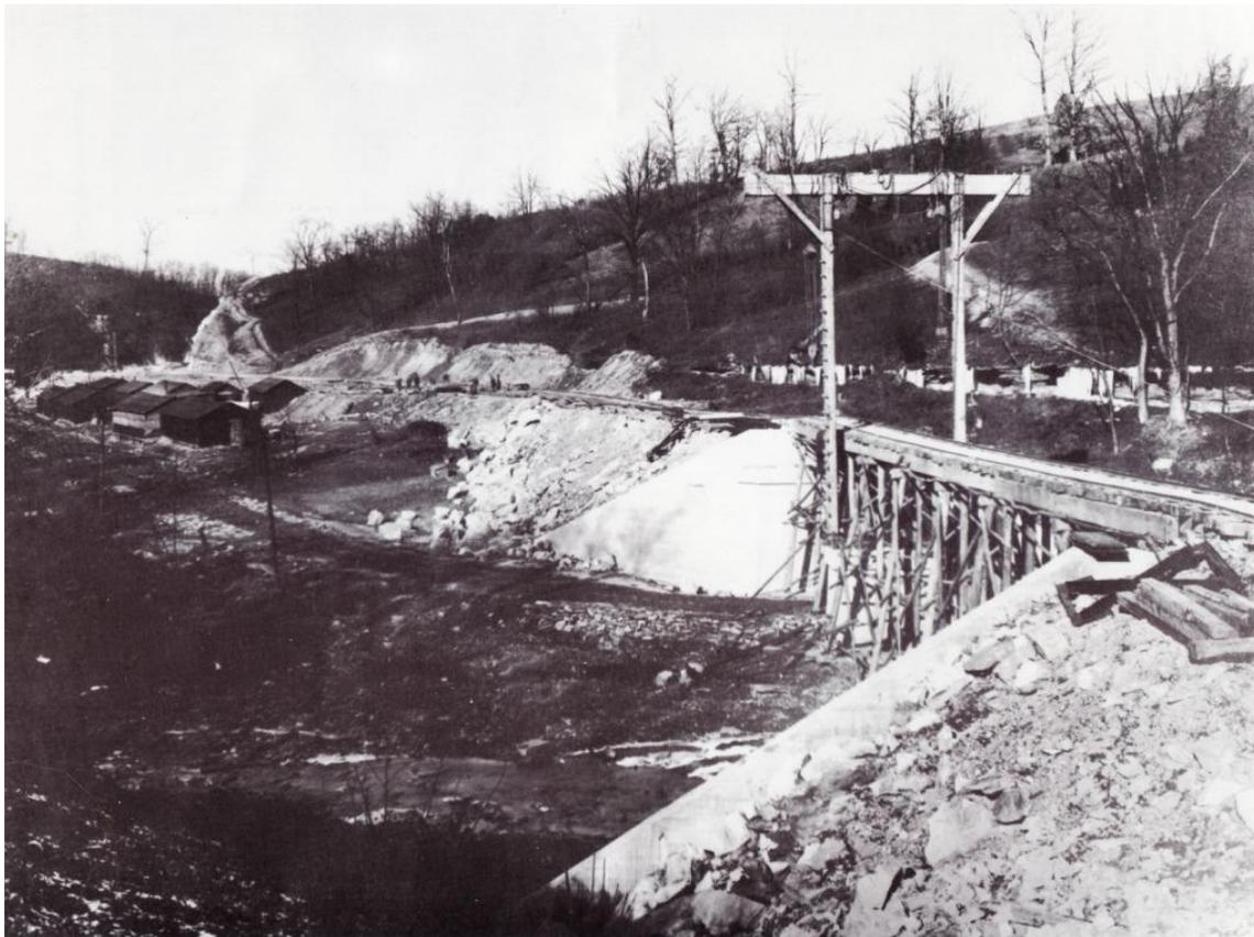
**A construction camp is seen at the east end of Montour Mine #4 as the railroad crosses Valley Brook Road in Peters Township. This temporary wooden trestle was used during construction of the railroad until a steel deck plate girder bridge could be built. Photo courtesy Dave Richards / Gene P. Schaeffer collection.**
