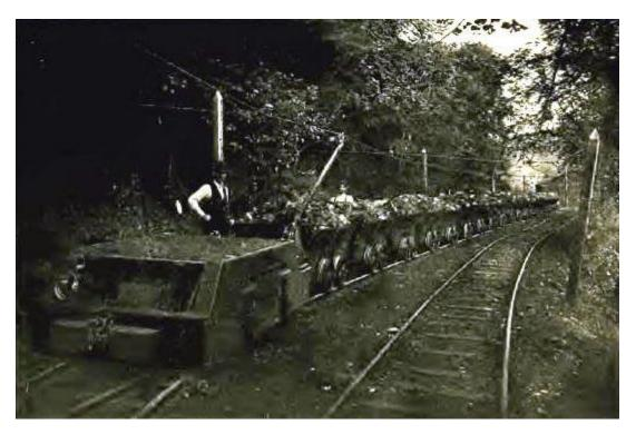
Another early view of the Moon Run tipple. This was taken when the mine first opened and had only one entry into the southern workings of the mine. Note the absence of electric poles and power plant, indicating the mine was cutting and hauling coal by hand and mules.
