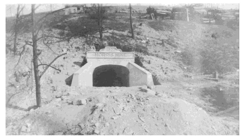
The sloped shaft portal is seen during construction in 1922. Mine tracks have not been laid and the slate dump which now covers the hillside is yet to be activated. Picture from Iva Mae Lose Hinton / Alan Hinton.
