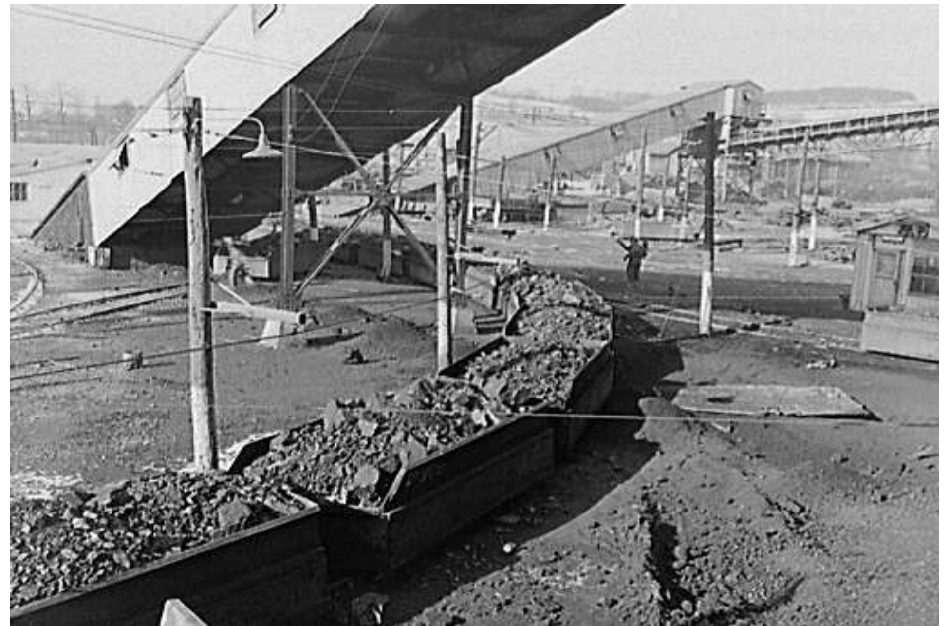
Loaded mine cars curve under the loading conveyor at the Westland tipple in 1942. Conveyors carrying slate and rock to the waste dump are seen in the background. John Collier, Jr. photo
